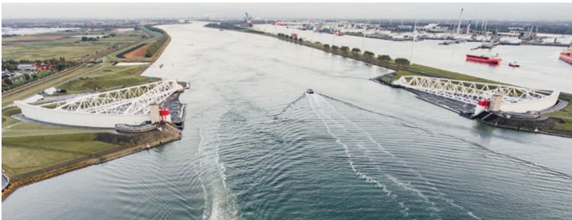
The Maeslantkering is one of the largest moving structures in the world. It closes off the waterway when water levels threaten to overflow the inland rivers. Each of its 'doors' is as tall as the Eiffel Tower (photo credits: Luca Locatelli).
